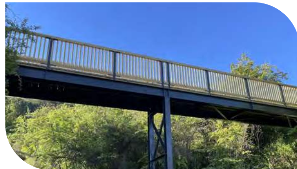
KUPERUS CROSSING 25m twin span bridged, hoisted into position at the end of 2023. The Kuperus Crossing was made possible thanks to the generosity of the Kuperus Family.
